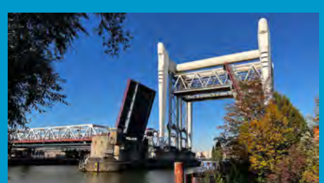
Replacement and renovation Traffic bridge
